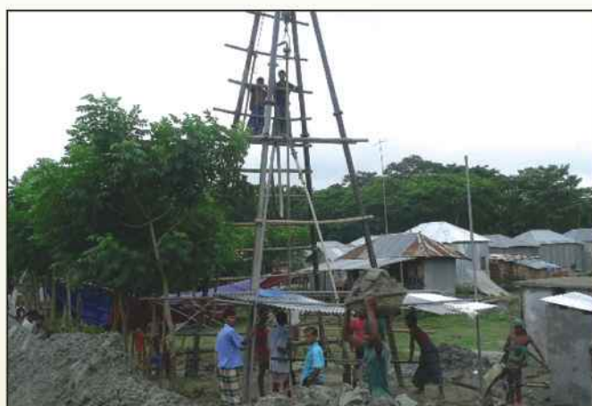
Deep tube well Installation system
